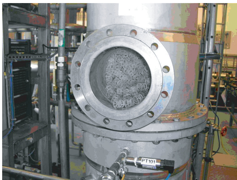
Fig. 5. Lower opening of absorption column in Kristianstad plant. The column is filled with pall rings. (Photo: R. Johansson.)
